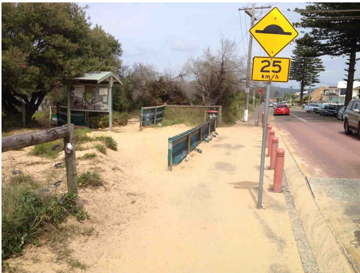
Figure 12 Sand Blowout at Barrenjeoy Rd Entrance - 2015
