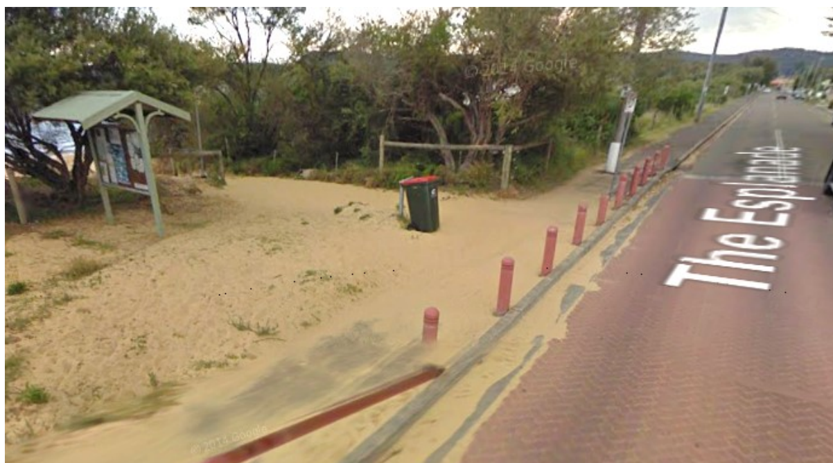
Figure 11 Sand Blowout at Barrenjoey Rd Entrance - 2009
